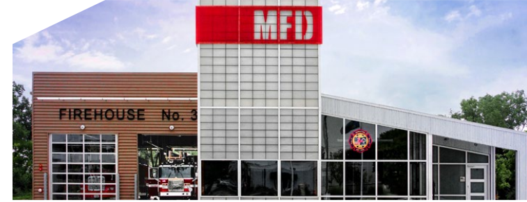
Manhattan Fire Station No. 3 - Manhattan, KS / Kalwall
