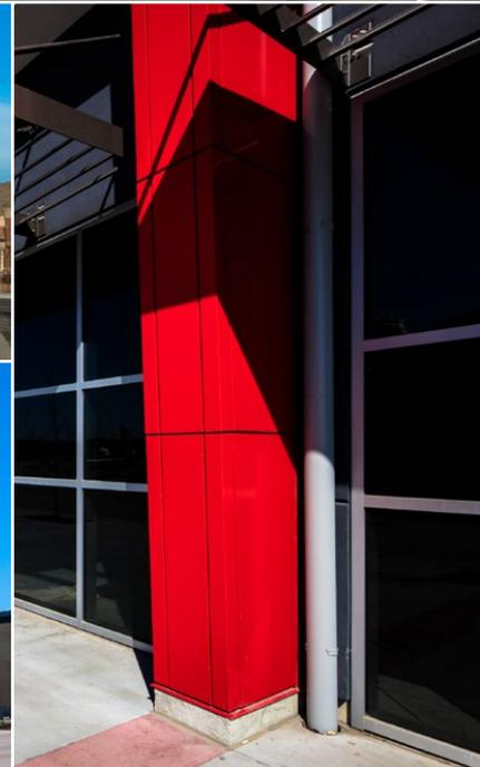
The Sieccoline metal panel system is a rear ventilated rainscreen wall system with variable joint sizes and an ease of installation that results in a clean and precise finished look using 4mm ACM (aluminum composite material).
